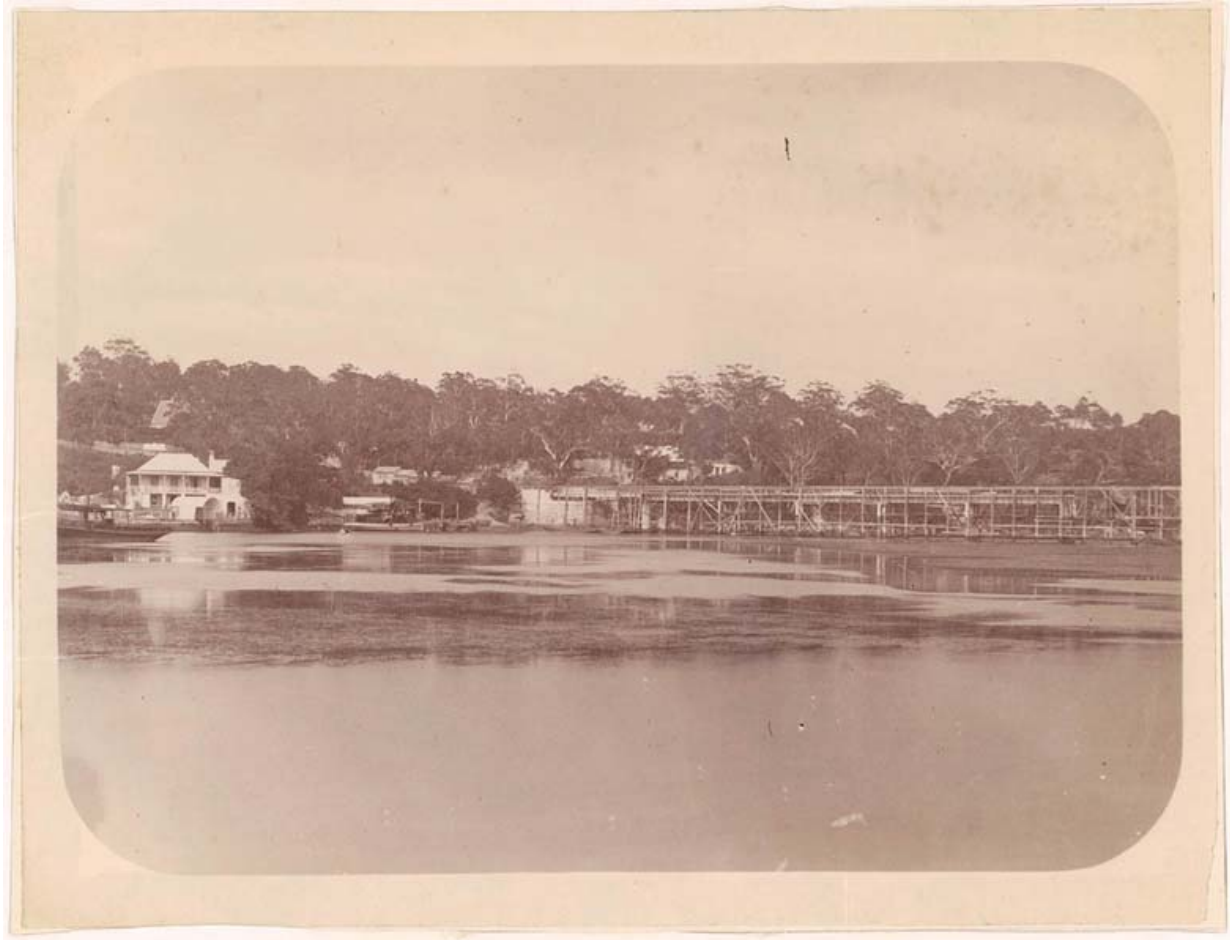
View of Fig Tree Bridge under construction, Lane Cove River, New South Wales. ca. 1874-1875
